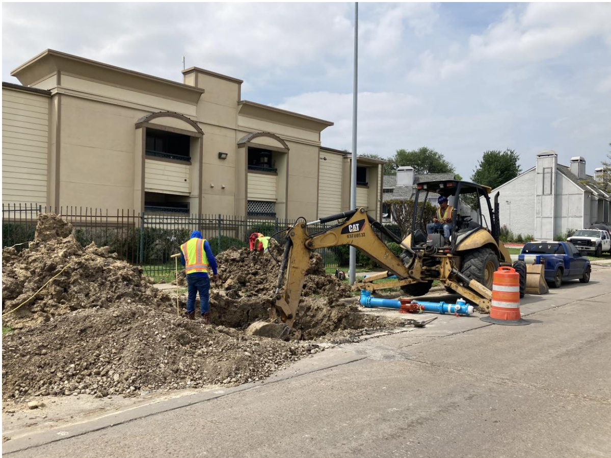
Installation of a fire hydrant on 12-inch water line.
