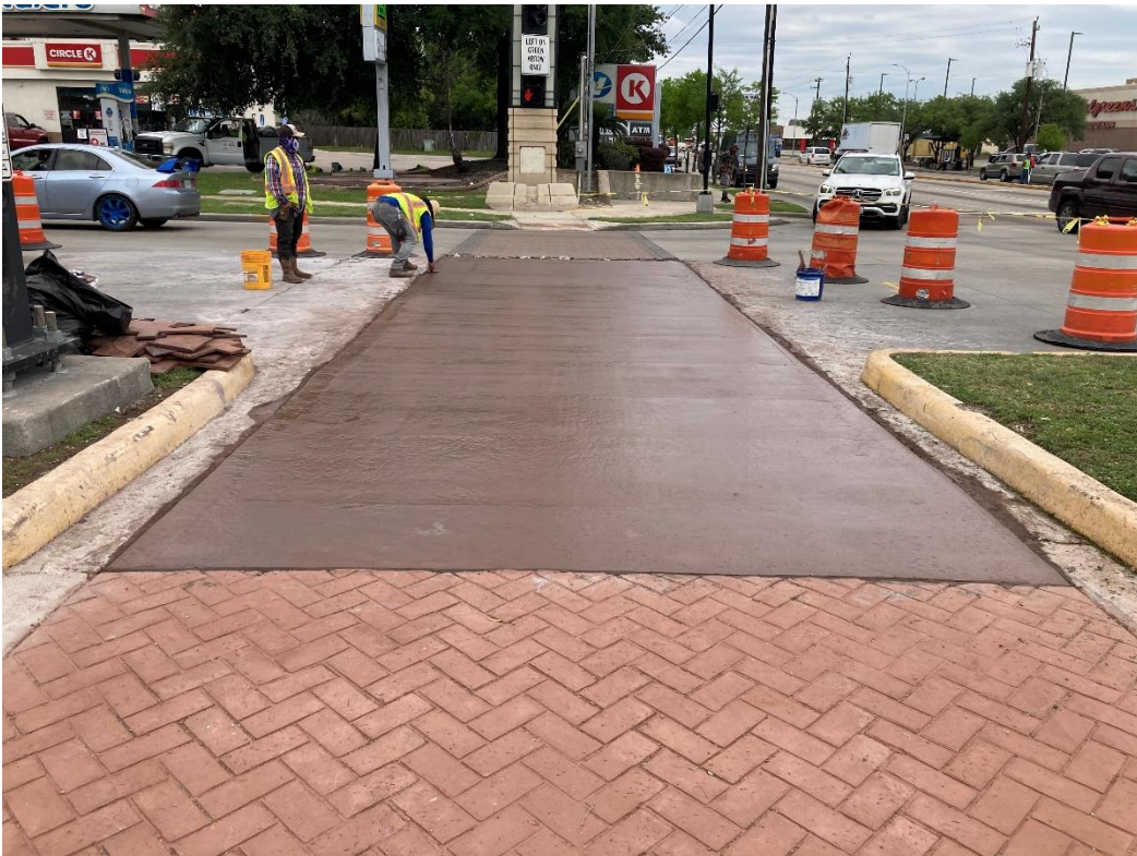
Finishing concrete prior to stamping.
