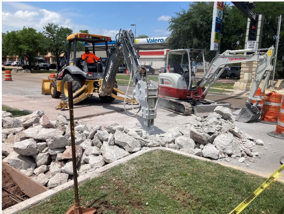
Removal of concrete pavement below existing paver crosswalk.
